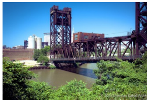
Columbus Road VERTICAL LIFT Bridge
