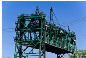
Eagle Avenue VERTICAL LIFT/VIADUCT Bridge
